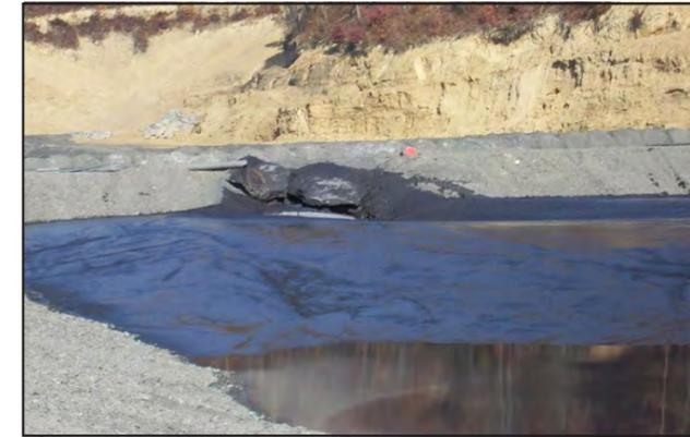
**Figure 3** – Slurry cell being filled with waste thickener underflow after OreBind Program treatment.
