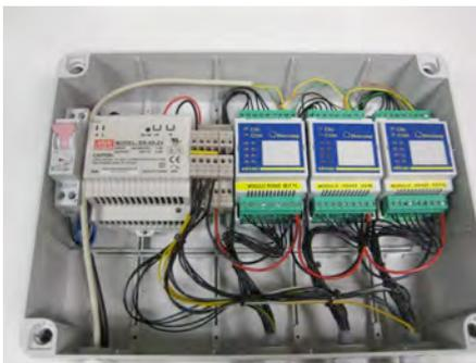
**Figure 2** – Splitter box used to manage signals between the RO trains and the 3D TRASAR unit.
