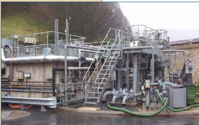
The high salinity feed upset the MBR sludge condition, causing excessive production of biopolymers and a consequential increase in membrane fouling. In addition, each time the saline levels rose significantly there was an associated substantial increase in foam levels.
