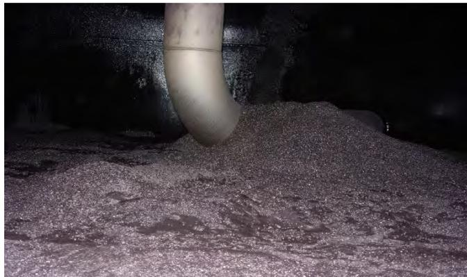
Figure 2 - Multi-media Filter after Backwash
