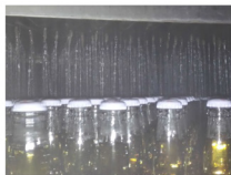
Mesh and nozzle are all unblocked resulting in uniform water flow distribution
